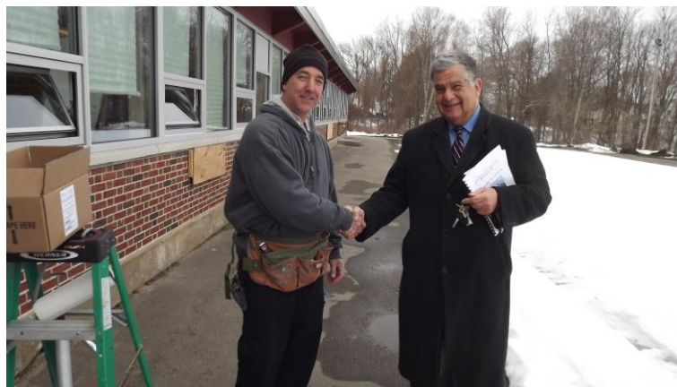
(L-R) Window installer and Mayor James J. Fiorentini at the Whittier School.
